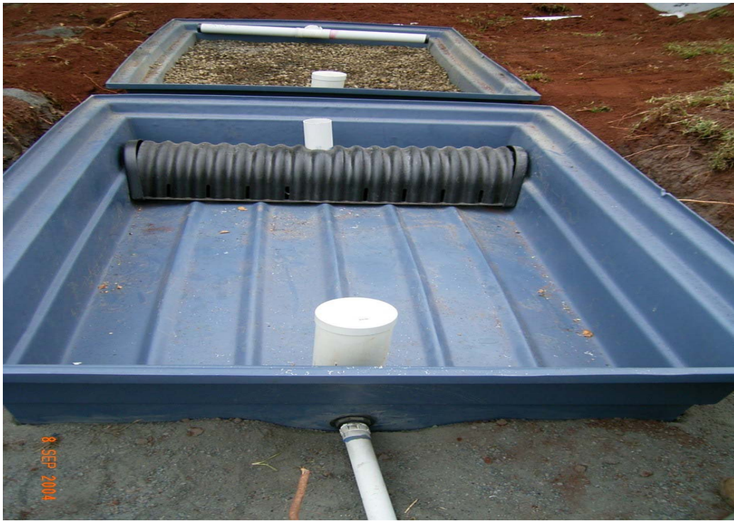
Duraplas Reed Bed Mould with an Arch Trenching Inlet. Moulds cost $390 And are the most popular membrane used for reed bed construction. Measures 3.1m long, 2m wide and 640mm deep.
