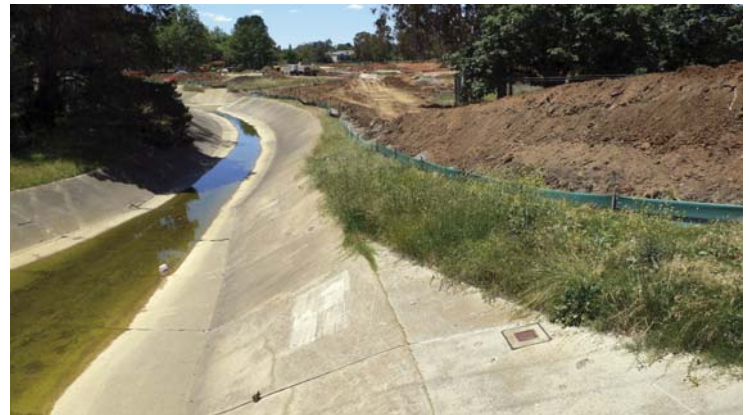
North Canberra Wetland Under Construction—Photo Paul Costigan
