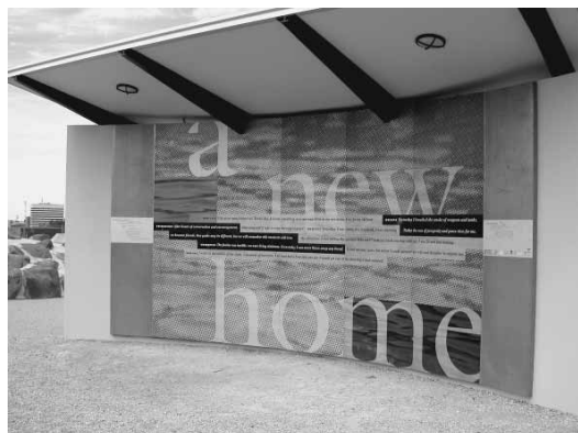
Migration Wall within North Hobart Cultural Park Tecton Projects, Hobart City Council
