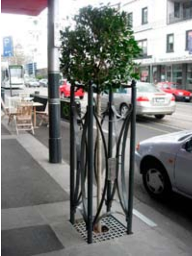
Figure 6 Glenferrie Road bioretention tree pits.
