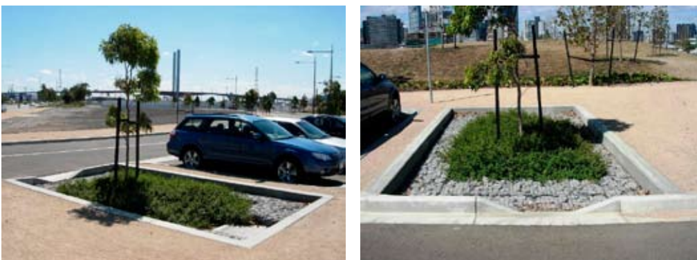
Figure 25 Docklands Point carpark rain garden
