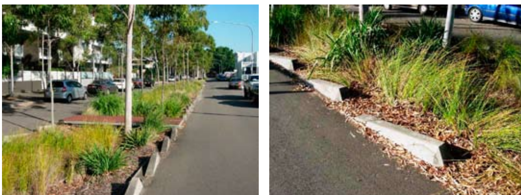
Figure 27 Victoria Park bioretention swale with permeable kerbing
