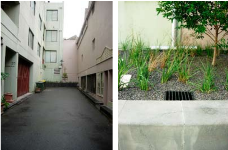
Figure 14 Davidsons Place rain garden
