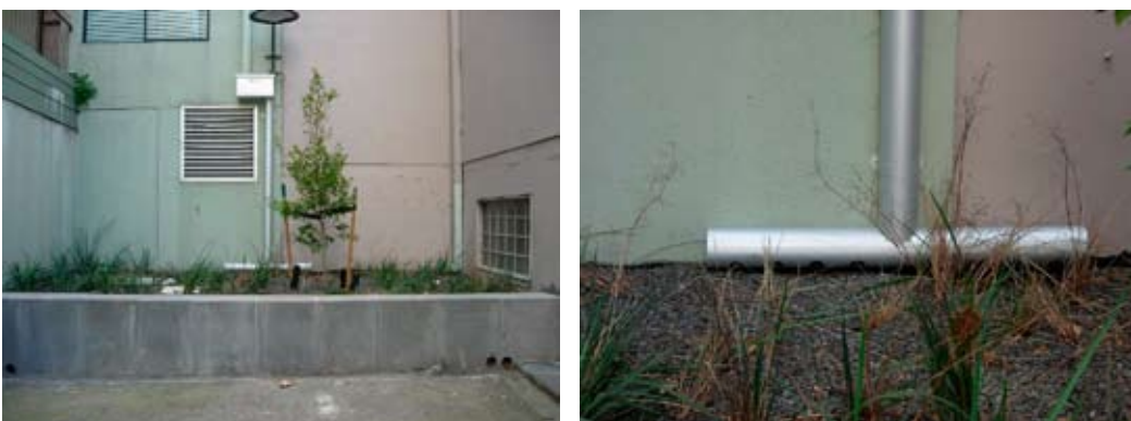
Figure 15 Davidsons Place rain garden
