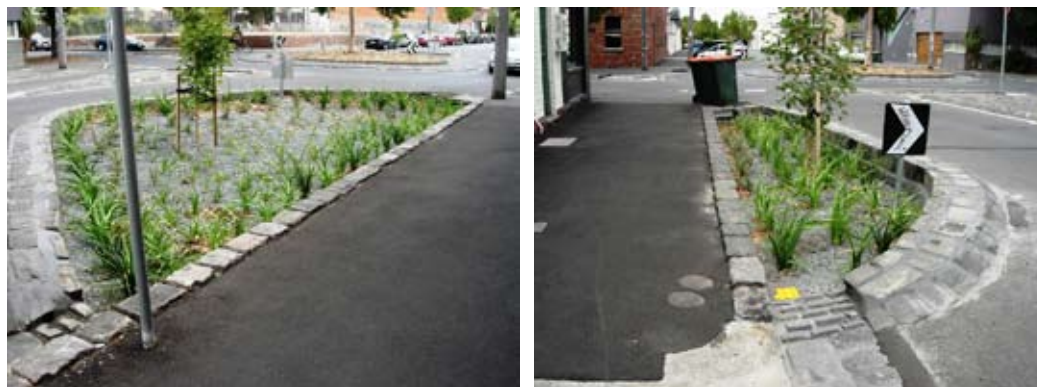
Figure 5 Napier Kerr Street rain garden
