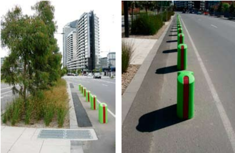
Figure 23 Batmans Hill Drive bioretention swale
