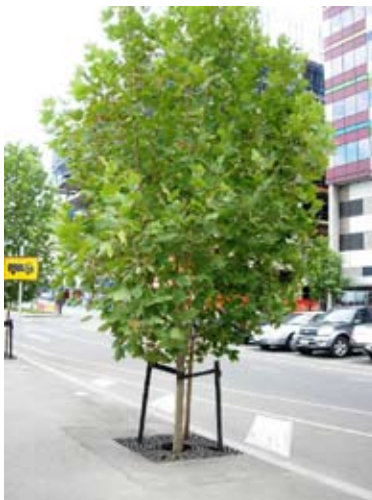
Figure 22 Bourke Street extension bioretention tree pits
