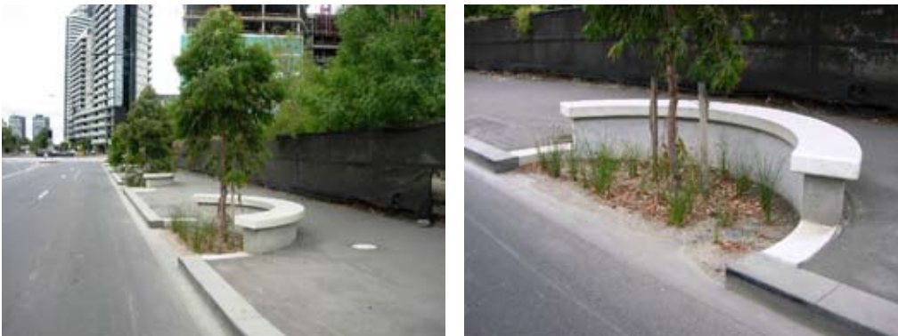
Figure 24 Batmans Hill Drive bioretention tree pits
