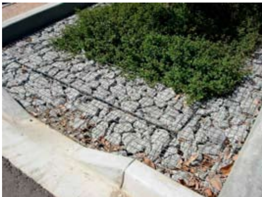
Figure 26 Docklands Point carpark gabion detail
