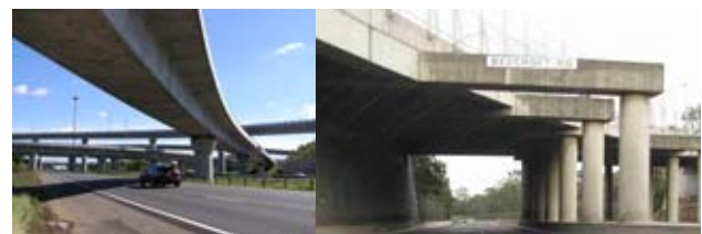
Plates 30, 31: Intriguing spatiality of motorway infrastructure, Sydney Australia, a.p. 2006
