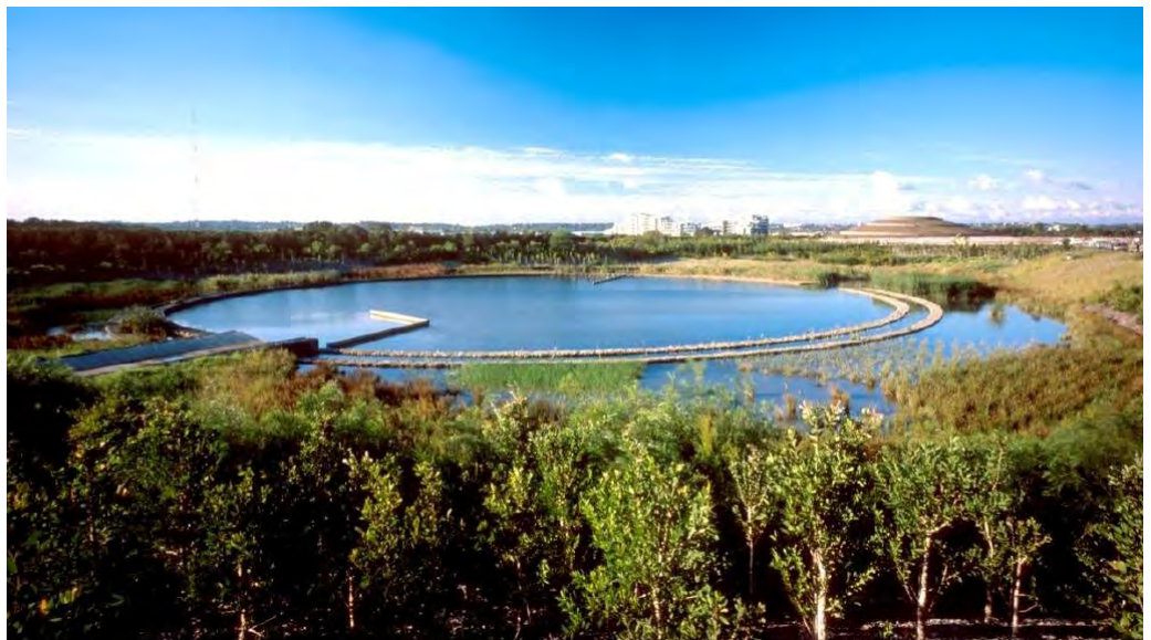
A feature of the parklands design was turning utilitarian components into elements of beauty. This water quality pond performs a variety of water purification and habitat functions as well as adding to the visual experience of the area.
