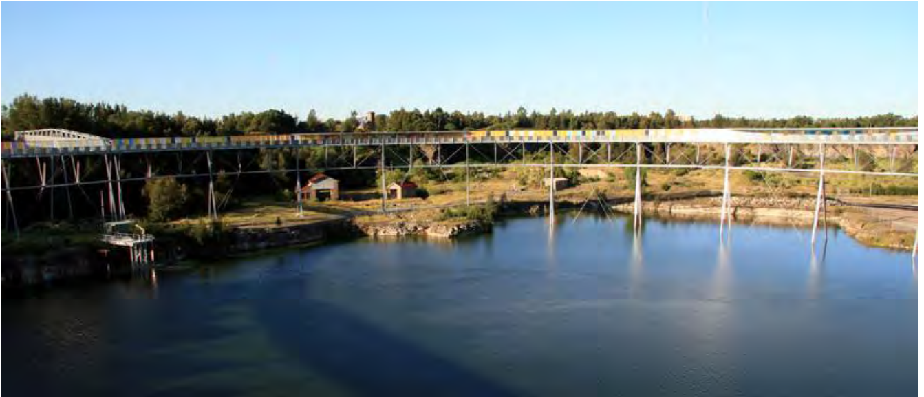
The Brick Pit ring is an inventive solution which provides access for people to experience this dramatic landform while protecting the primary habitat of the Green and Golden Bell Frog.
