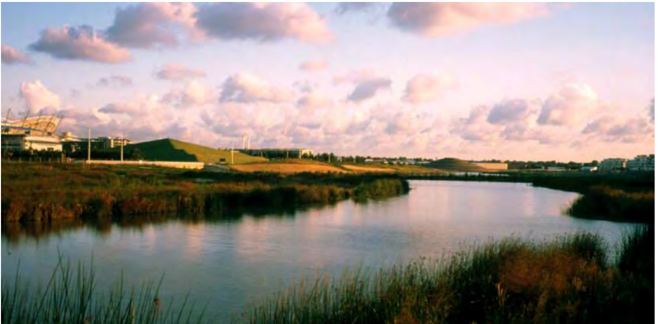
Haslams Creek following restoration of the sinuous creek from and wetlands in 2000 was the first stage of the parklands construction.
