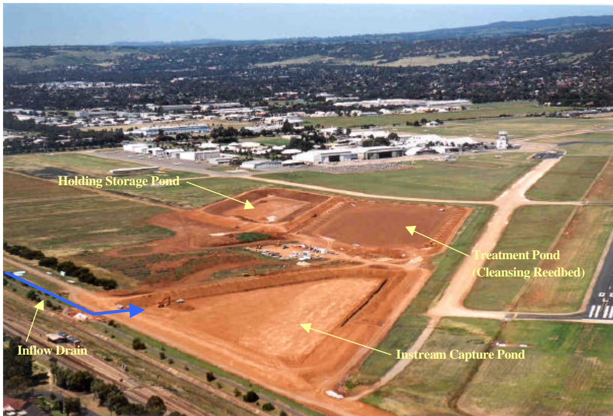
Aerial view of the construction work in progress at Parafield Airport
