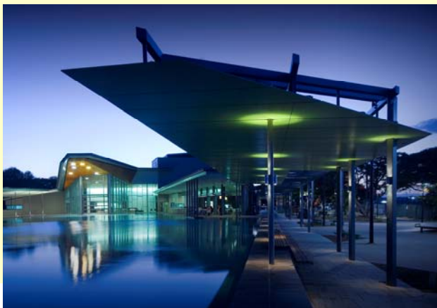
Thuringowa Riverway Commendation for Design in Landscape Architecture 2007 AILA QLD Project Awards (Photograph: Christopher Frederick Jones)
